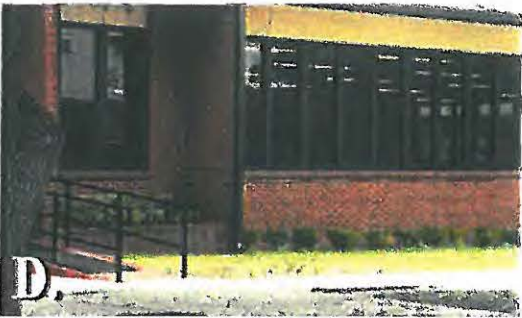
Energy efficient window upgrades throughout the campus.
