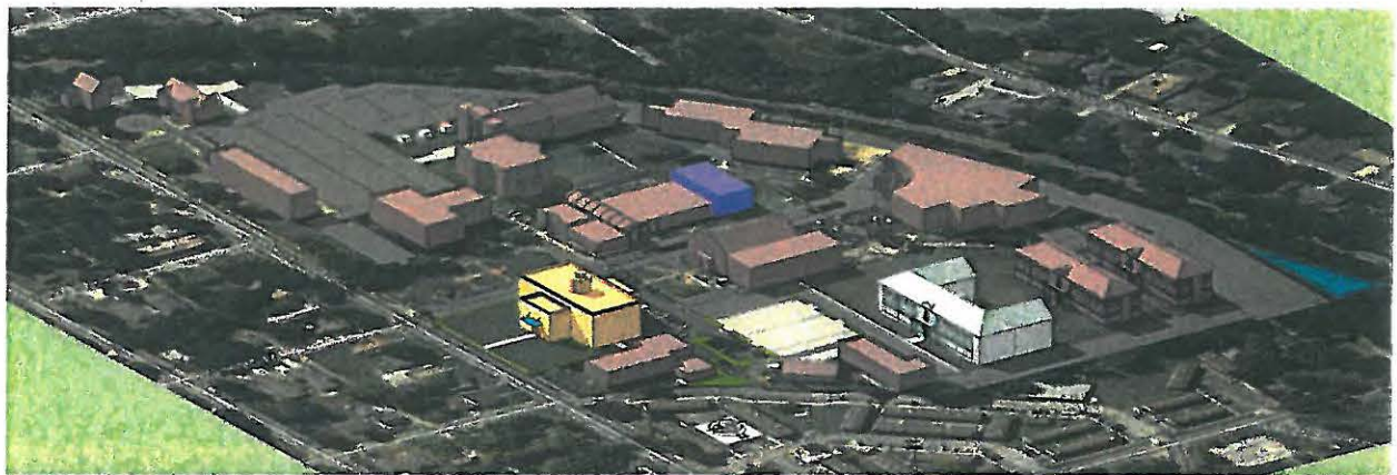
PHASE IV NORTHEAST VIEW
